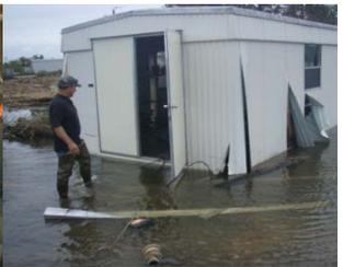
**Figure 10:** Portable Storage Shed #2 at Galva Canal that was raised three feet to avoid flooding.
