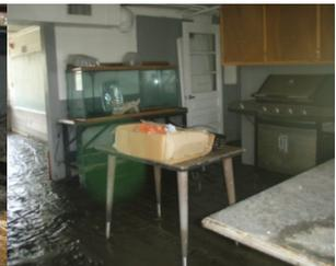
**Figure 8:** Two-three inches of silt on ground floor of Turtle Cove lodge.
